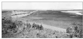
3–24 & 3–25 Dykes in Grand Pré are still topped with vegetation from the salt marshes. Rock facing is currently used to help withstand the force of the tides, rather than the wooden plank facing that was common in the 19th century.
